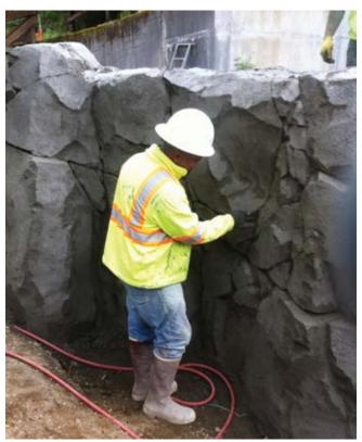
Fig. 4: Shotcrete finishing for bedrock textures
