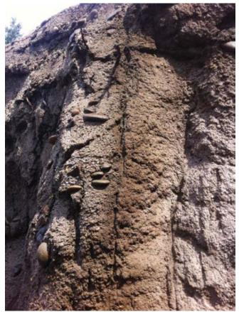
Fig. 2: Earthen textures with embedded cobbles, roots, integral pigments, and topical stains
