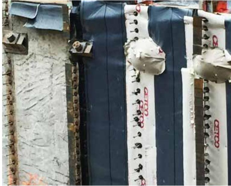
Fig. 3: Form-and-pour requires far more form tie anchor penetrations in the blindside waterproofing than reinforcing bar stabilization for shotcrete
