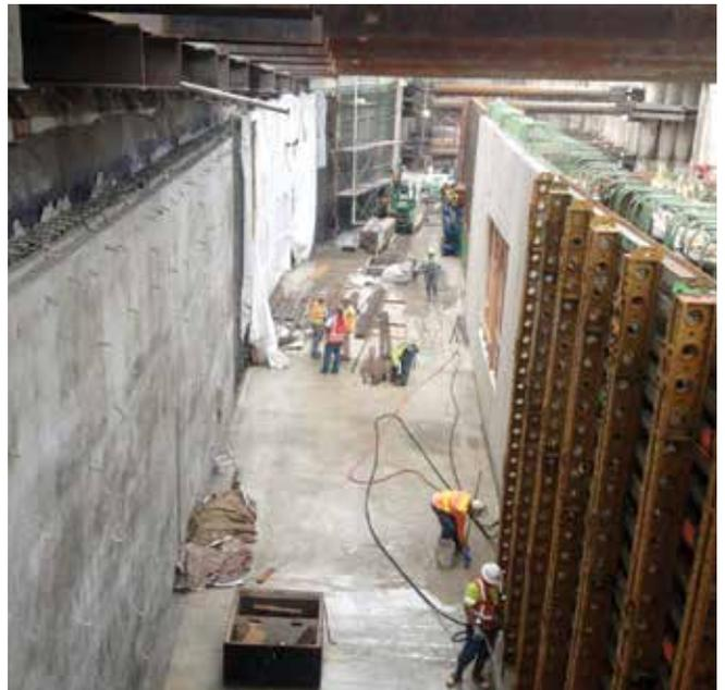
*Fig. 5: Large highway tunnel project in Seattle, WA, with over 750,000 ft<sup>2</sup> (69,677.28 m<sup>2</sup>) of structural shotcrete, completely done with a post-injected hydrophilic membrane/textile composite system for blindside waterproofing*
