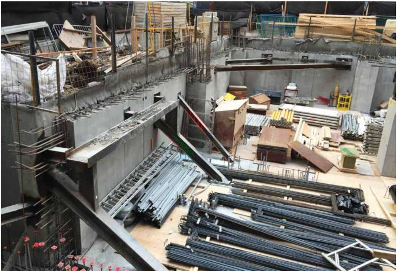
Fig. 1: Downtown high-rise hospital, below-grade blindsided walls, with shoring rakers and densely reinforced high-strength pilasters supporting 20 floors
