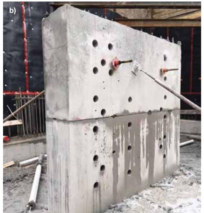
Fig. 2(a) and (b): Honeycomb and voids in form-and-pour (left) and dense sharp-edged structural shotcrete (right)
