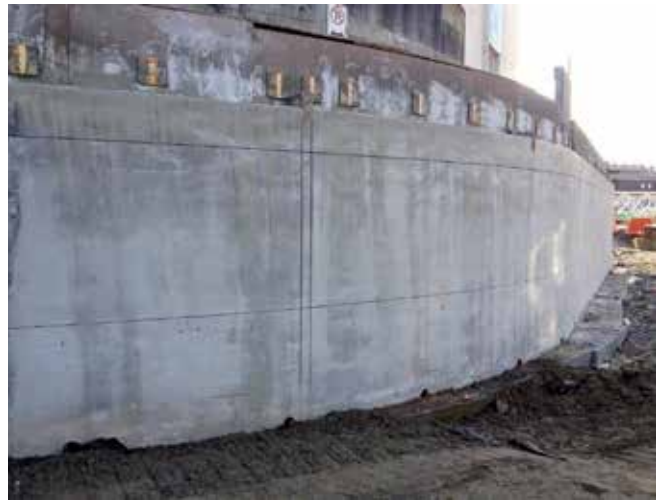
Fig. 9: Finish troweled curved wall, with post saw-cut architectural reveals
