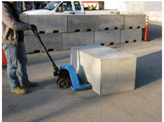
Fig. 10: Rebound and waste shotcrete cast onsite into useable retaining wall and barrier blocks, further contributing to the sustainability of shotcrete
