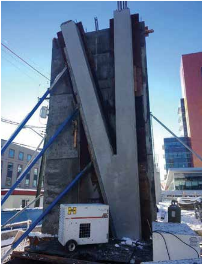
Fig. 3: Complex forming for architectural “Y” columns, using one-sided shoot panels
