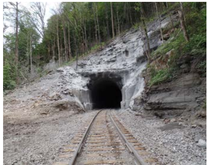
Fig. 8: East portal—final liner
