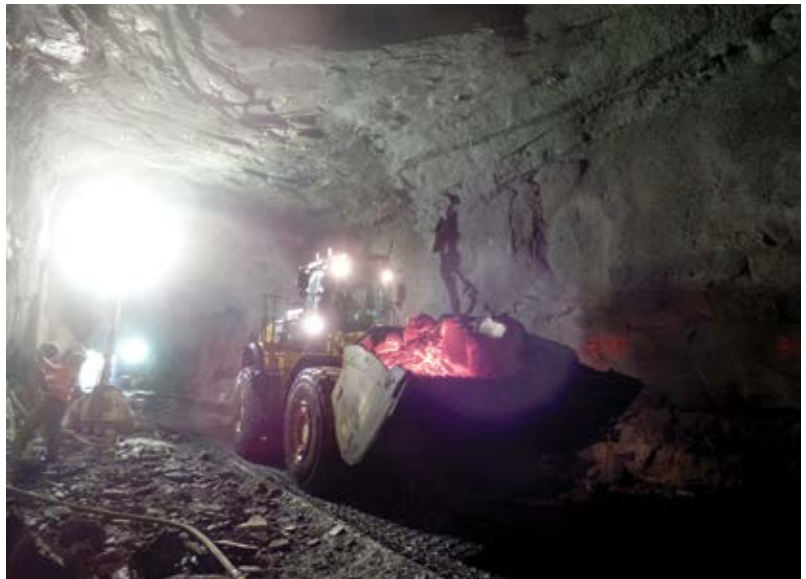
Fig. 3: Muck removal with loader
