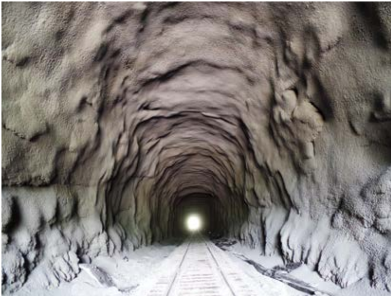
Fig. 6: View of final liner from west portal
