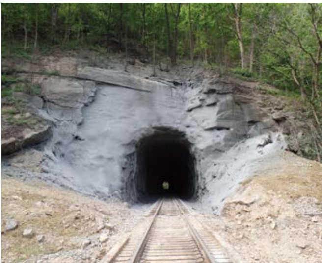
Fig. 7: West portal—final liner
