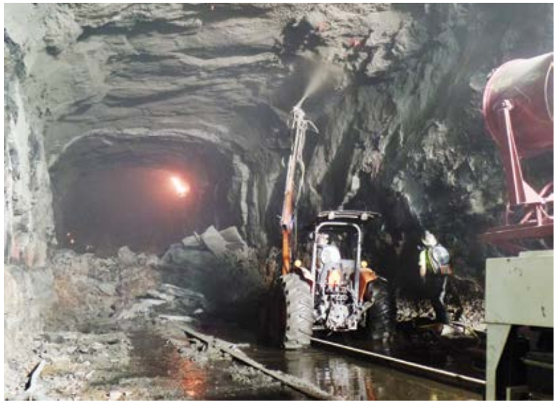
Fig. 2: Initial shotcrete roof support
