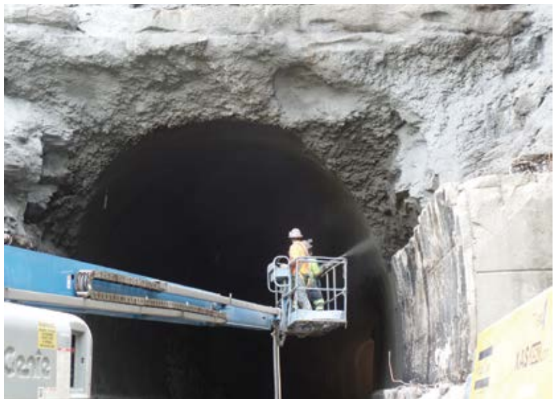
Fig. 4: ACI Certified Nozzelman applying shotcrete to east portal
