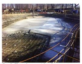
Fig. 5: Floor shotcrete (placed in stages)
