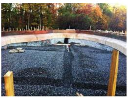
Fig. 3: Plumbing system under shotcrete shell
