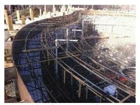
Fig. 4: Steel reinforcement on radius steps
