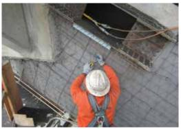
Fig. 4: Repairing mesh prior to shoot
