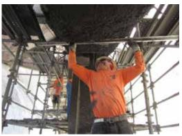
Fig. 8: Overhead finishing
