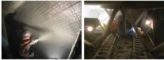
Fig. 2 and 3: Shotcrete placement inside the arches
