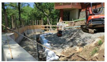
Fig. 7: Extensive formwork required for cast-in-place concrete
