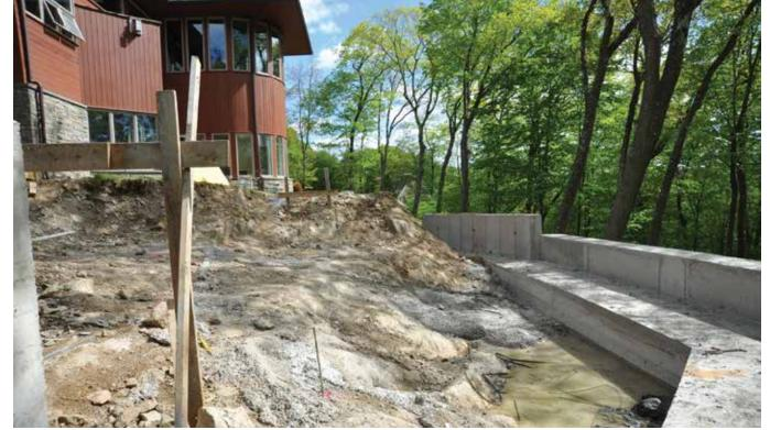
Fig. 5: Cast-in-place concrete footing to support pool structure
