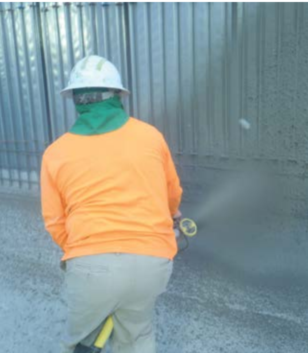
Fig. 2: Exterior shotcreting from the ground
