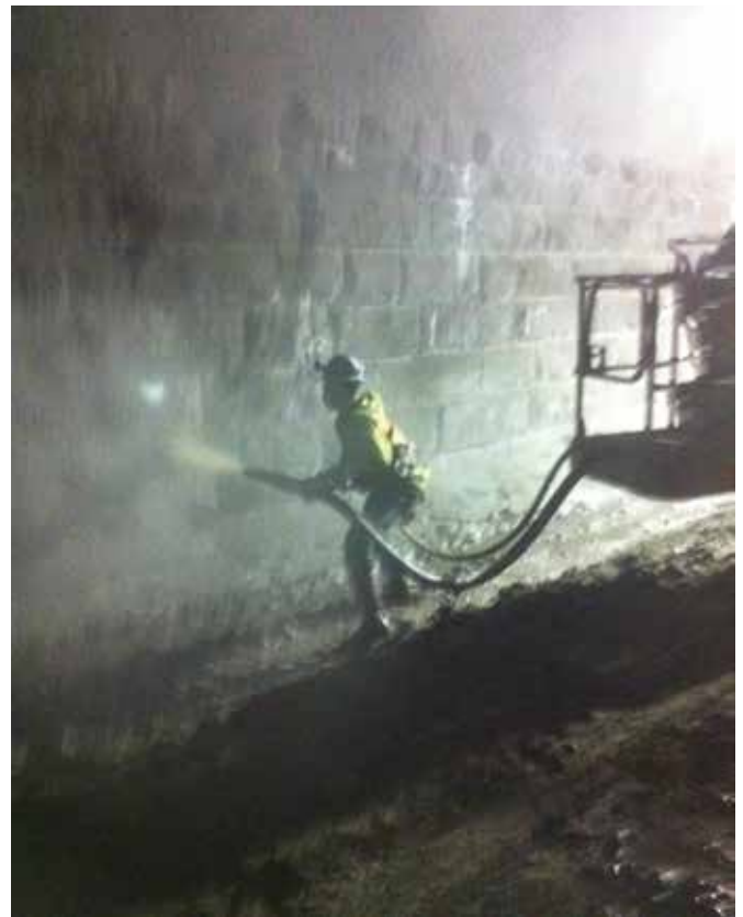
Fig. 2: Nozzlemen placed 100 bags of shotcrete a day, sometimes working on steep slopes
