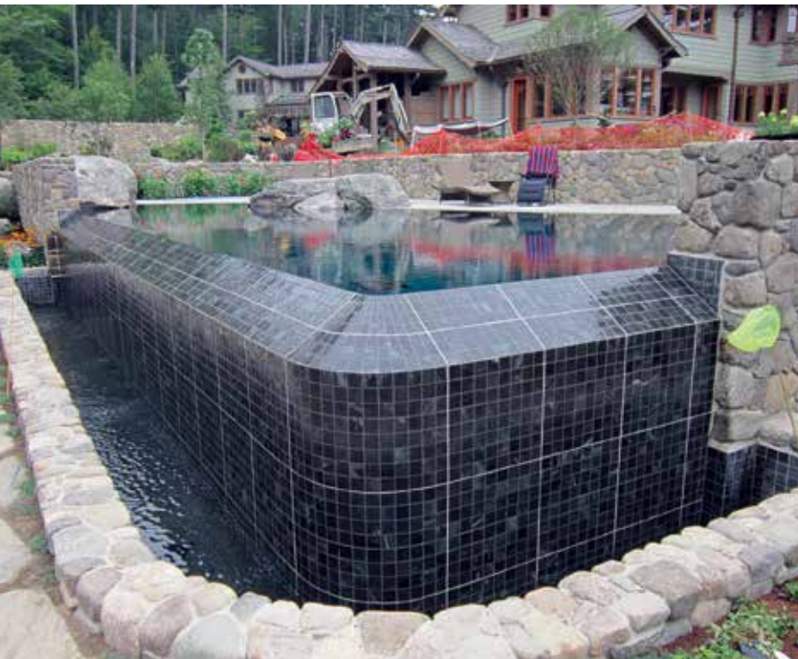
Fig. 6: Completed pool from the negative-edge side
