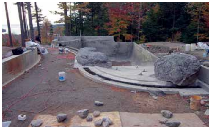
Fig. 4: Completed shotcrete with large rocks placed
