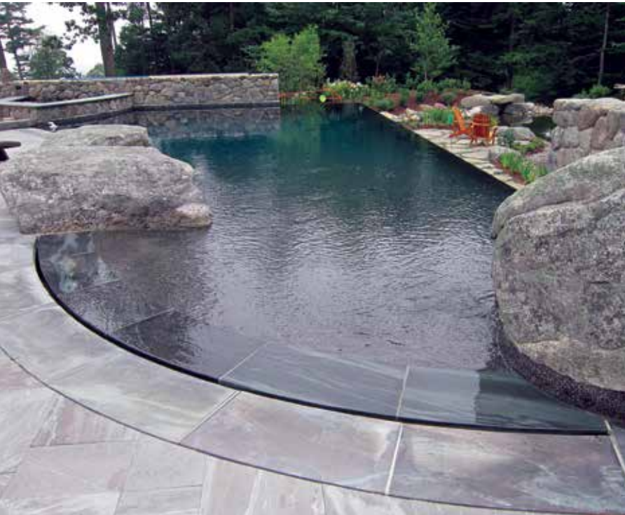
Fig. 5: Completed pool from the beach-entry end
