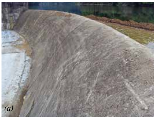
Fig. 1: Deterioration before rehabilitation: (a) spillway; and (b) wall
