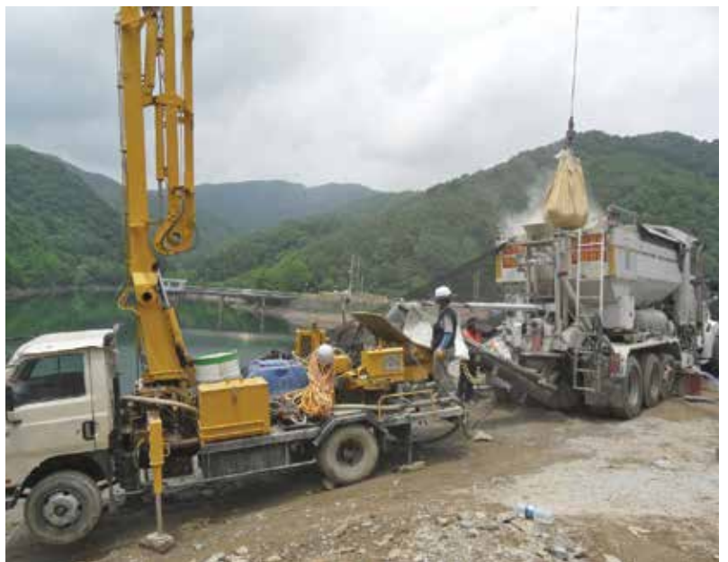
Fig. 3: A mobile mixer supplying concrete to the shotcrete pump
