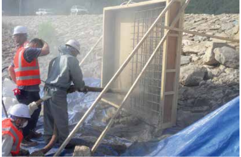
Fig. 5: Mockup panel test
