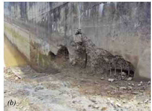
Fig. 1: Deterioration before rehabilitation: (a) spillway; and (b) wall
