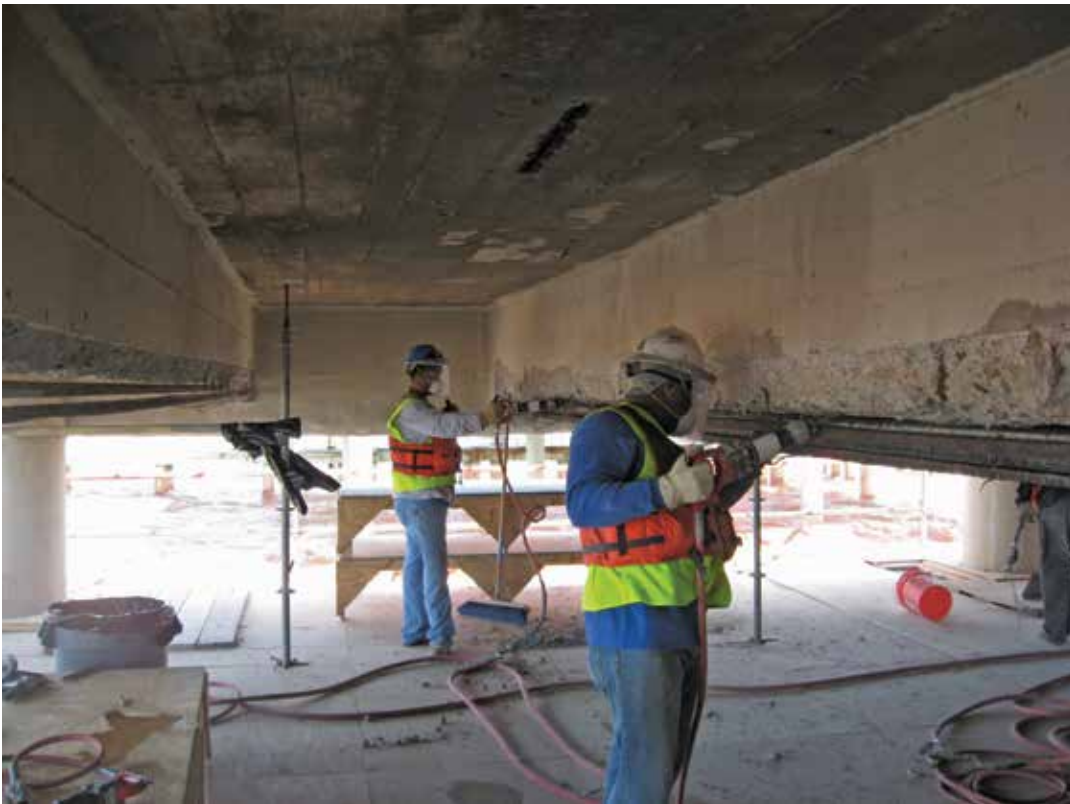
Fig. 2: Surface preparation of deck support beams
