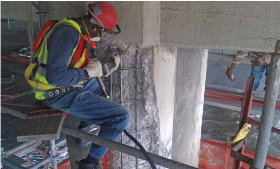
Fig. 3: Surface preparation of pier columns
