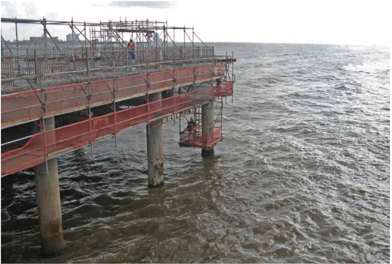
Fig. 4: Scaffolding setup for open access to underside of deck
