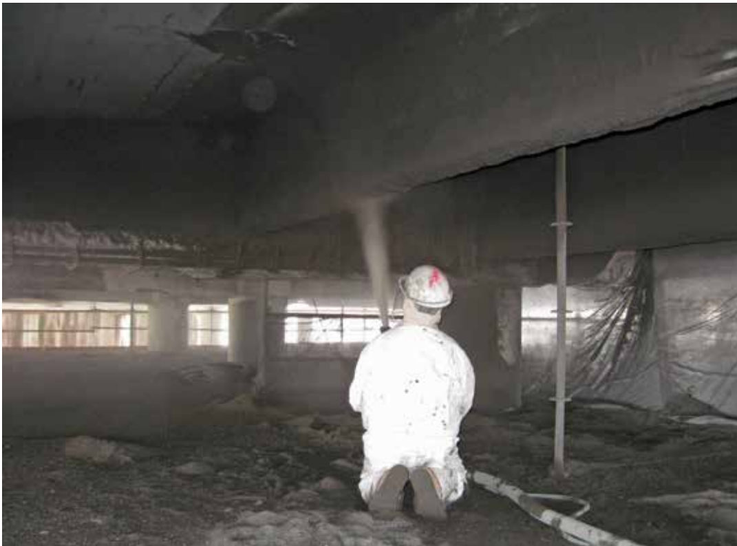
Fig. 5: Shotcreting deck beam overhead with very limited access height
