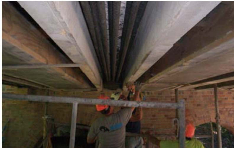
Fig. 5: Finishing the beams
