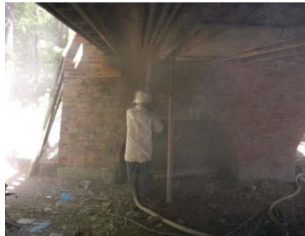
Fig. 3: Placement of shotcrete under confined working conditions
