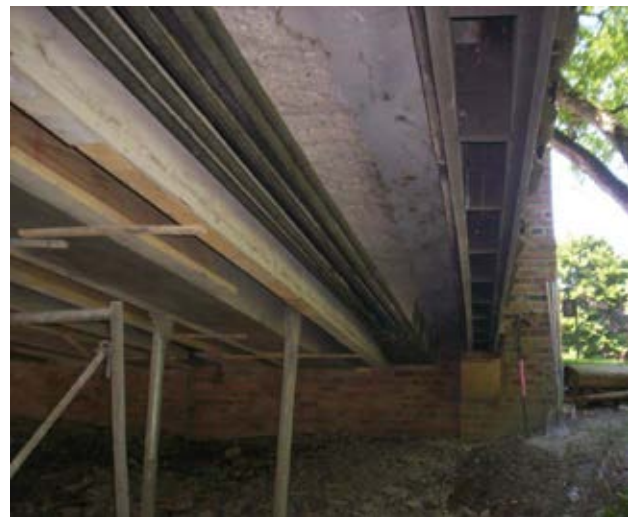
Fig. 2: Underside of bridge prepared for repair
