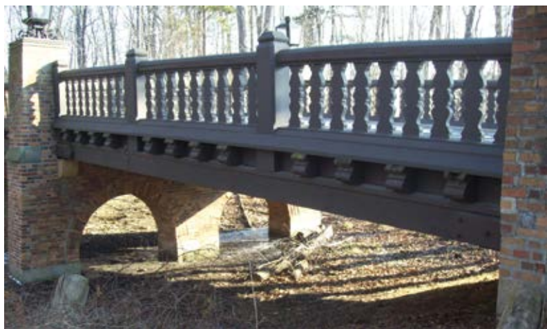
Fig. 6: Oakland University's Meadow Brook Hall Bridge
