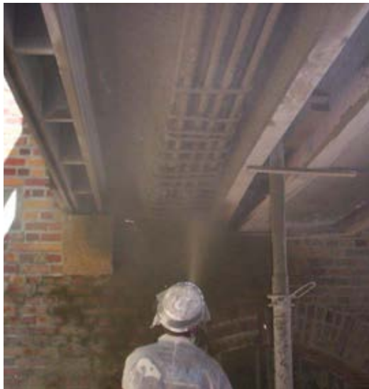
Fig. 4: Close-up of shotcrete placement
