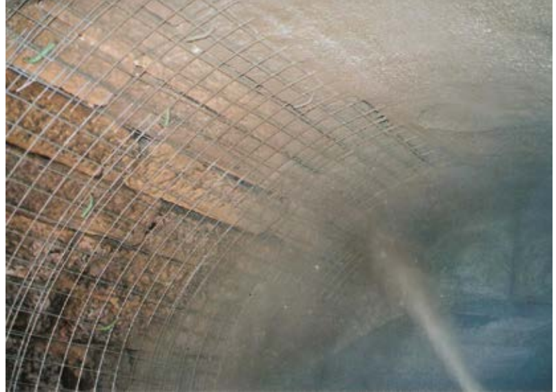
Fig. 5: Dry-process shotcrete being gunned overhead in an underground culvert
