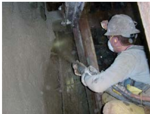
Fig. 3: Application of shotcrete on shaft wall
