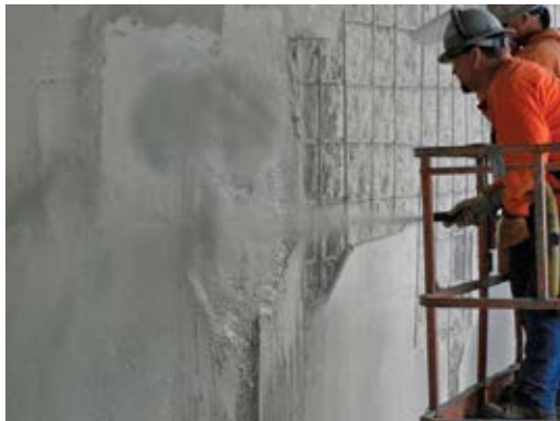
Fig. 1: Shotcrete repair on bridge abutment using low-permeability, rapid-setting cement
