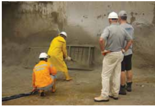
Fig. 4: Nozzleman participating in the vertical performance examination
