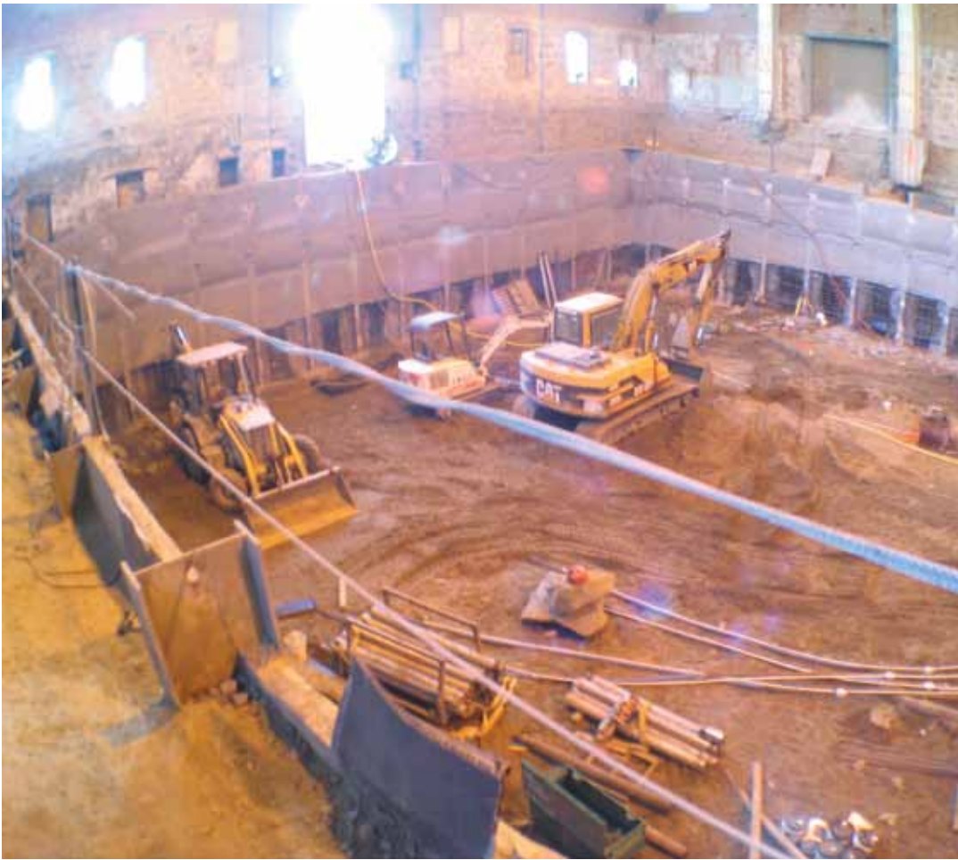
Fig. 3: Shotcrete soldier pile shoring
