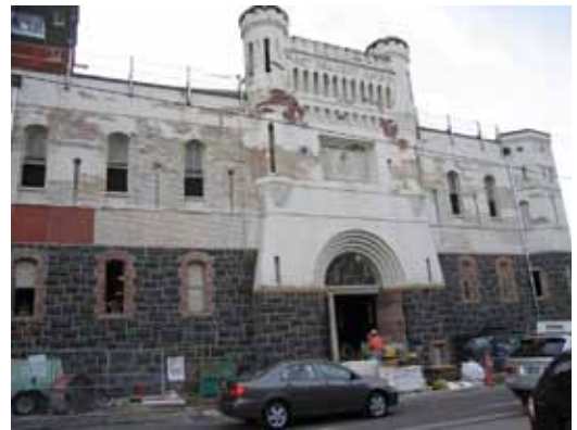
Fig. 7: Outside during renovation
