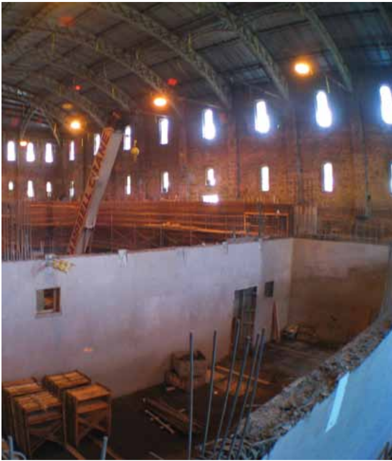
Fig. 5: Shotcrete after stripping forms
