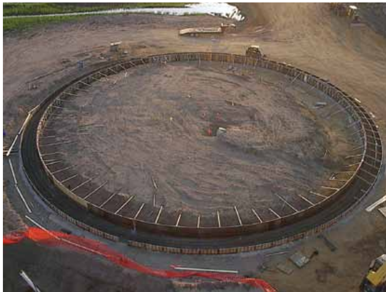
Fig. 1: Construction of a typical dome foundation
