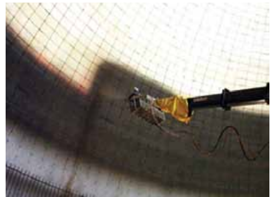
Fig. 3: Shotcrete is applied in layers
