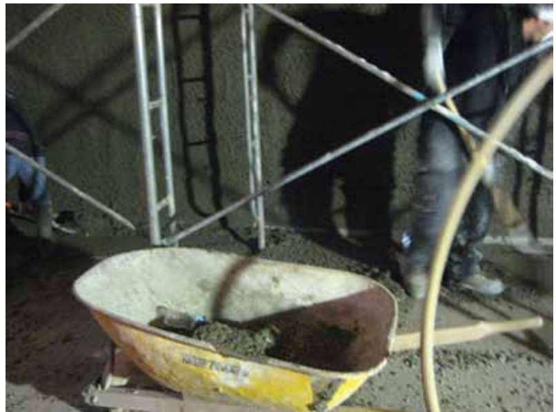
Fig. 4: Rebound materials collected and used as backfill materials
