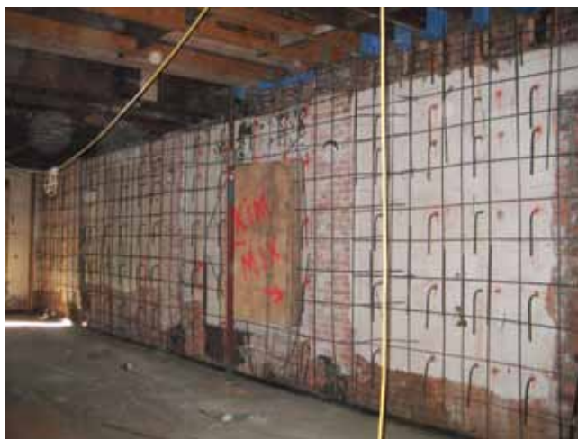
Fig. 2: Shotcrete applied to a masonry wall for seismic retrofit for a heritage building in Vancouver, BC, Canada
