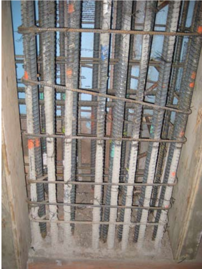
Fig. 12: View of reinforcing bar in splice zone at bottom of pilaster
