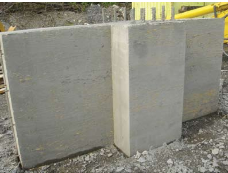
Fig. 6: Stripped back-face of shotcreted pilaster mock-up. Note good consolidation of shotcrete
