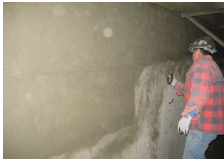
Fig. 11: View of a wall being finished
