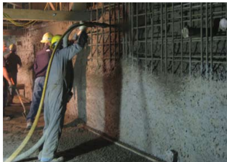
Fig. 9: Shooting of a wall using the bench gunning technique
