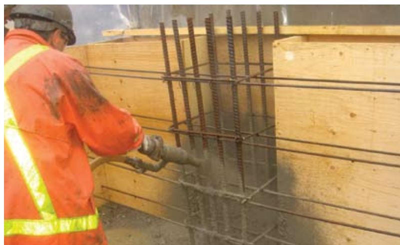
Fig. 5: Shooting pilaster mock-up
