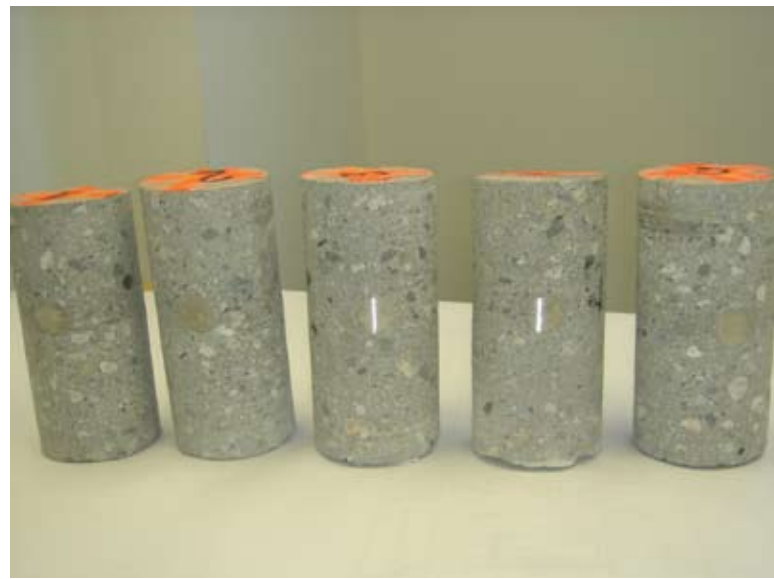
Fig. 7: Cores extracted from reinforcing bar locations in pilaster mock-up—all core Grades 1 or 1.5
