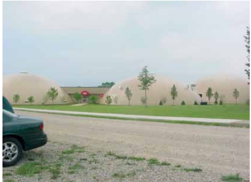
Valley R-6 School District in Caledonia, MO, already has three monolithic dome buildings—two classroom domes and a multipurpose facility (pictured here). It is now building two new 85 ft (26 m) diameter dome structures on the same site. One dome will house five classrooms, whereas the other will feature three classrooms and a large library and media center. The new domes will unite students from kindergarten through grade 12 on the same campus
