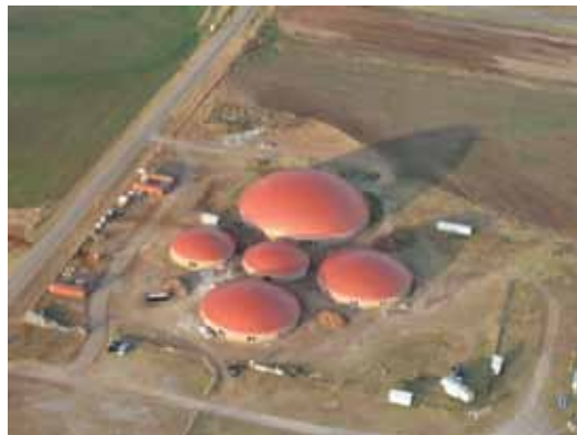
This is an aerial view of the newest monolithic dome school in Oklahoma. Construction is nearing completion on a new middle school and high school in Geronimo, consisting of five modular monolithic domes
