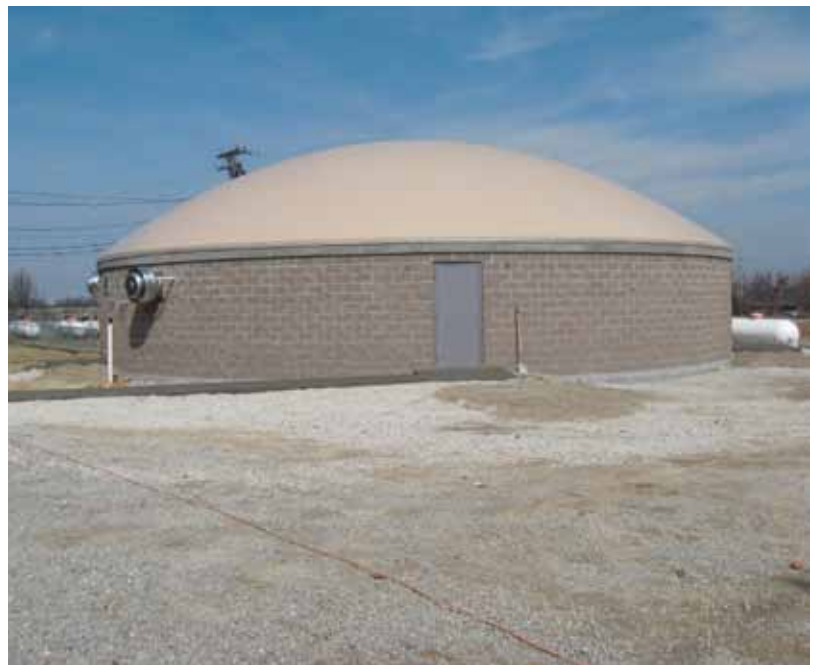
This 2700 ft 2 (251 m 2 ) monolithic dome preschool building in the Niangua R-V School District in Missouri was financed by a FEMA predisaster mitigation grant of $313,000 designed to cover 90% of the construction costs for a new building. Completed in April 2009, the dome replaces a nearby double-wide trailer that school officials concede was a tornado magnet
