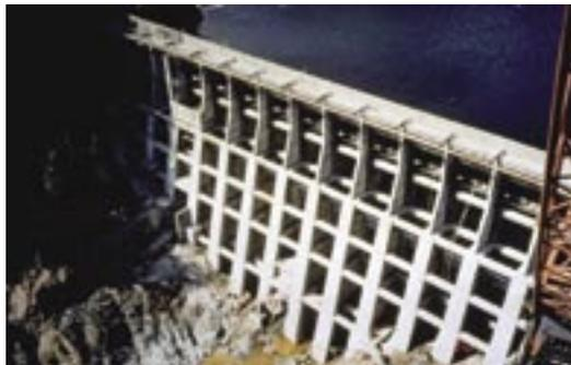
*Fig. 11: Shotcrete repairs to upper buttresses, Jordan River Dam*
