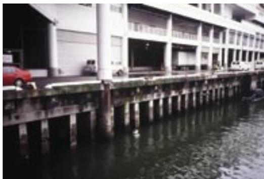
*Fig. 1: Dry-mix shotcrete repaired beams at Canada Place*
