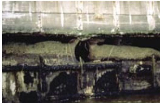
Fig. 2: Typical deterioration in 60-year-old berth faces at Port of Saint John, New Brunswick, caused by frost, alkali aggregate reactivity, and tidal/wave action
