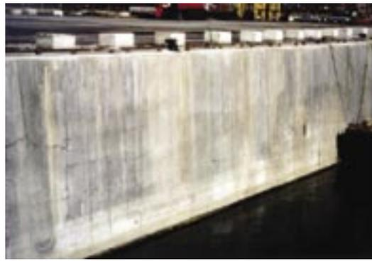
Fig. 5: Portion of the completed wet-mix shotcrete repairs to berth face at the Port of Montreal
