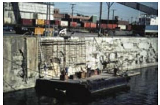
Fig. 4: Removal of deteriorated berth face concrete at Port of Montreal, Quebec
