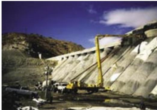
*Fig. 10: Seismic retrofit of the upstream face of the Littlerock Dam*
