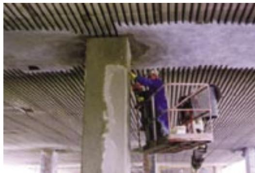
Fig. 13: Shotcrete repairs to Metropolitan Boulevard, Montreal, Quebec
