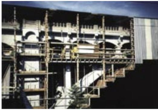
*Fig. 12: Shotcrete repaired Depoe Bay Bridge with thermal-sprayed zinc anode cathodic protection coating*
