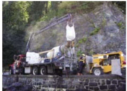
Fig. 7: Shotcrete "train" on the Stanley Park Seawall, Vancouver, BC
