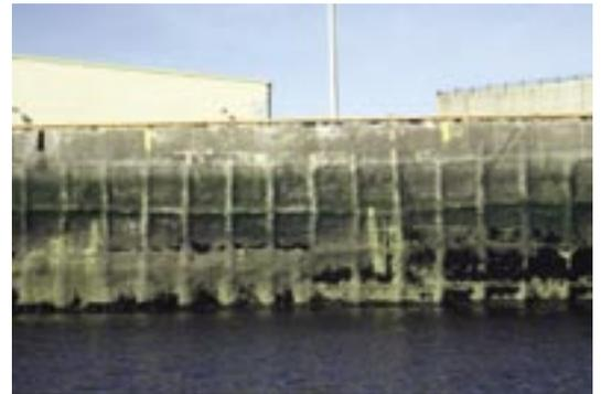
Fig. 3: View of shotcrete repaired berth faces at the Port of Saint John after 10 years in service and over 2000 freezing-and-thawing cycles
