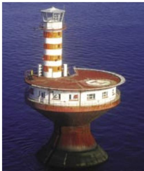
Fig. 6: Haute-Fond Prince Lighthouse in Gulf of St. Lawrence, Quebec, after completion of shotcrete repairs
