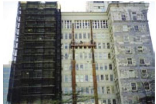
Fig. 16: Shotcrete repair of heritage building, Vancouver, BC
