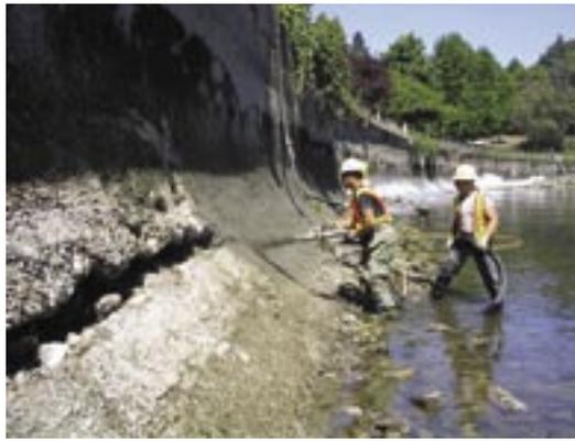
*Fig. 9: Shotcrete repairs to damaged concrete-faced rip-rap in the Devonian Park part of Stanley Park Seawall*
