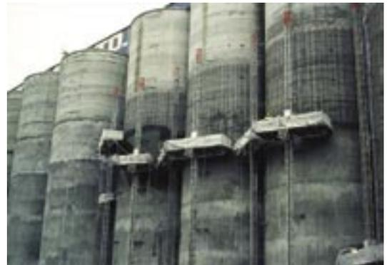
Fig. 14: Shotcrete strengthening of grain silos at Prince Rupert, BC
