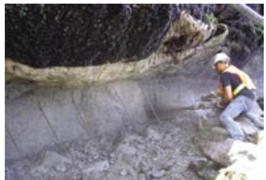
Fig. 8: Underpinning of a cave under the seawall near Siwash Rock, Stanley Park Seawall, Vancouver, BC, using macrosynthetic fiber-reinforced wet-mix shotcrete
