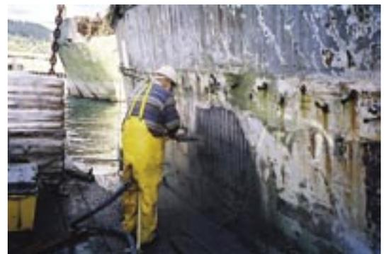
Fig. 15: Shotcrete repaired floating concrete ships, Powell River, BC
