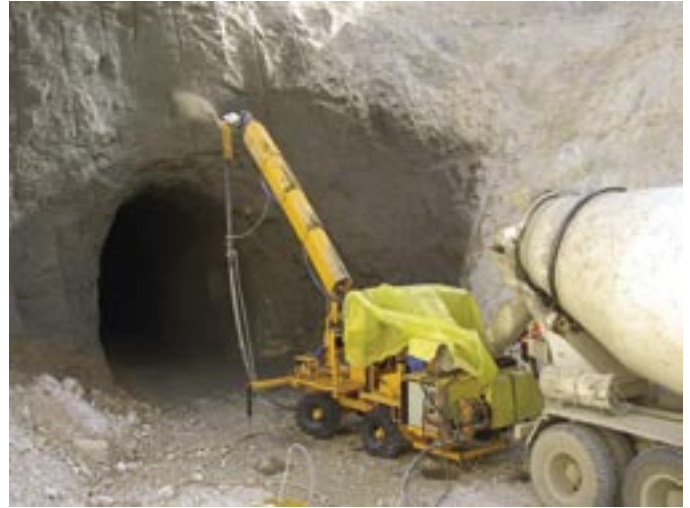
Tunnel portal—robotic shotcrete application
