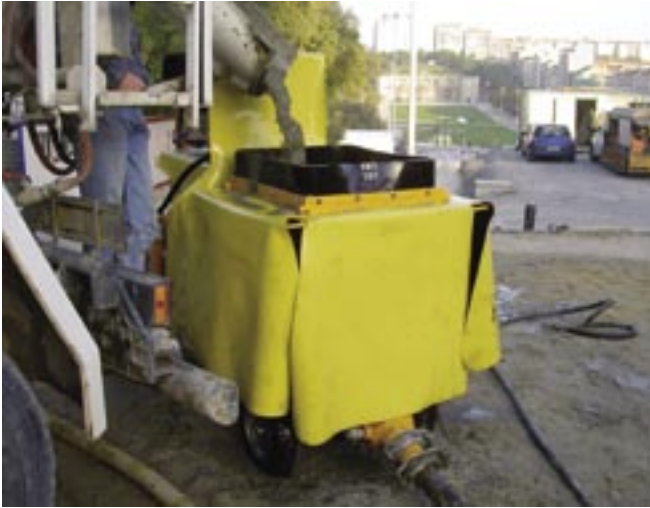
Wet/dry-shotcrete machine—rotary barrel type (continuous feed)
