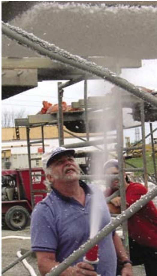
Fig. 4: Application of cellulose
