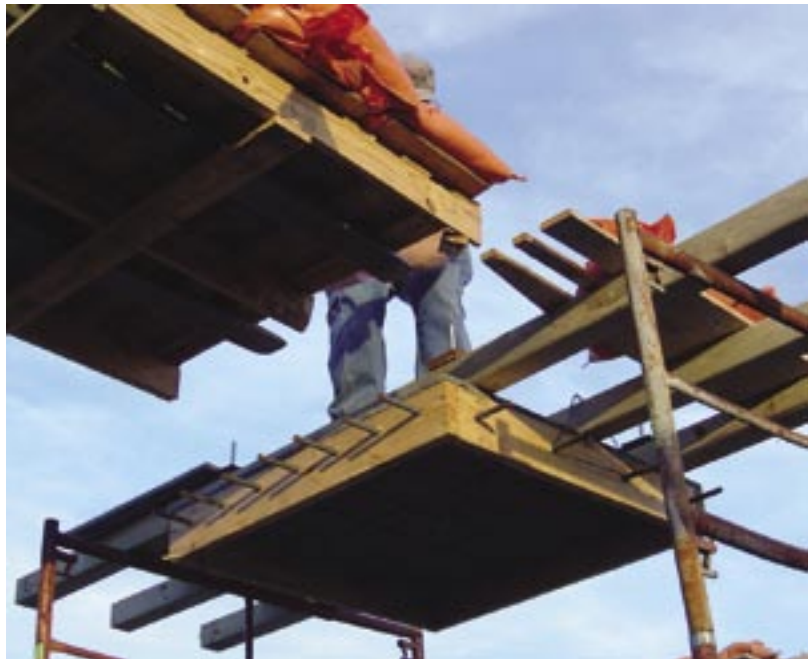
Fig. 2: Scaffolding used to support the test panels
