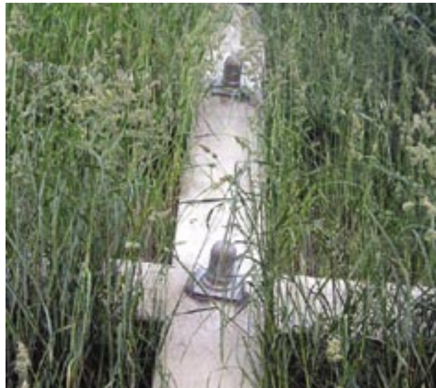
Fig. 5: Grid Beam covered with grasses
