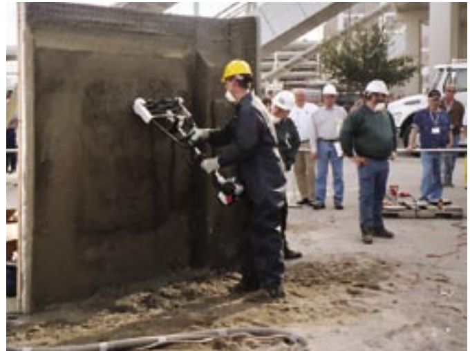
Striking-off the repaired section
