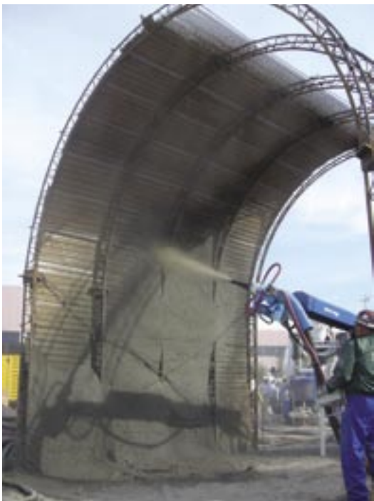
A tunnel mock-up was shot with a robot
