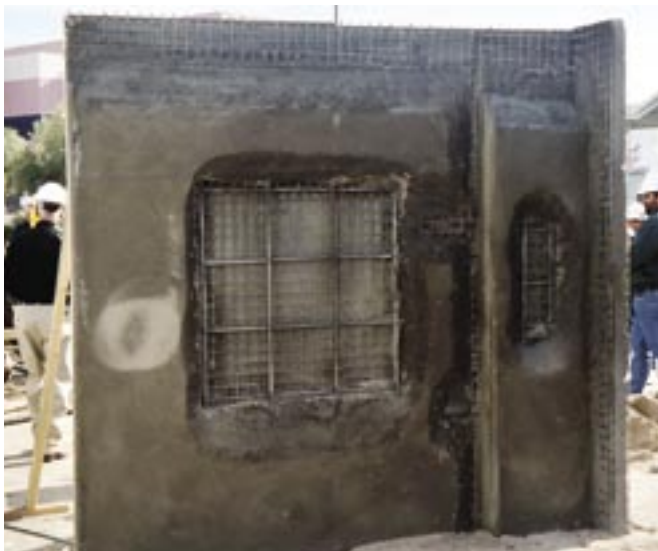
Ready for shotcrete repairs
