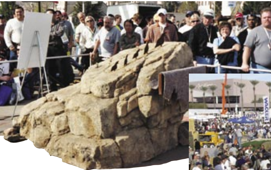
A shotcrete rockscape was constructed
