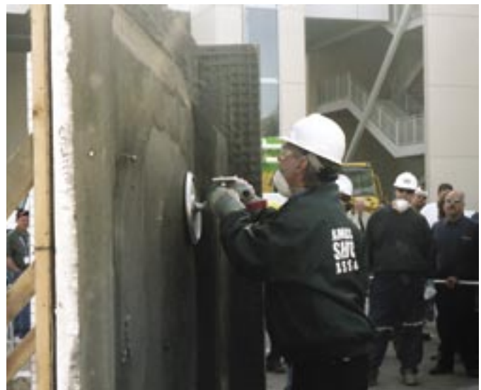
Finishing the repaired section
