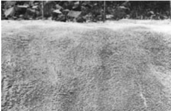
Colored shotcrete transition with natural rock slope
