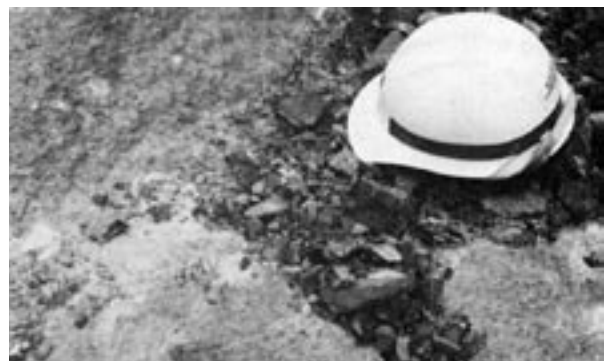
Colored shotcrete with rock fragments of natural material
