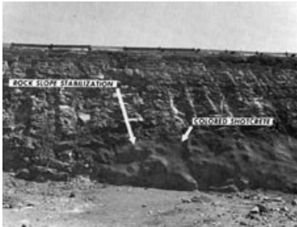
Fig. 3: Ririe Dam right abutment stabilization
