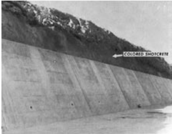
Fig. 2: Ririe Dam Spillway channel
