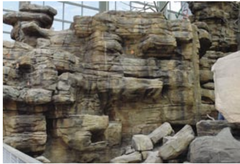
Shotcrete rockwork formations rising to a level of over 80 ft above finish floors also camouflage mechanical ducts and vent openings
