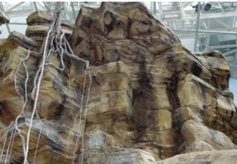
Shotcrete artificial rockwork cliffs combined with artificial vines and roots resemble water-worn canyons of Australia
