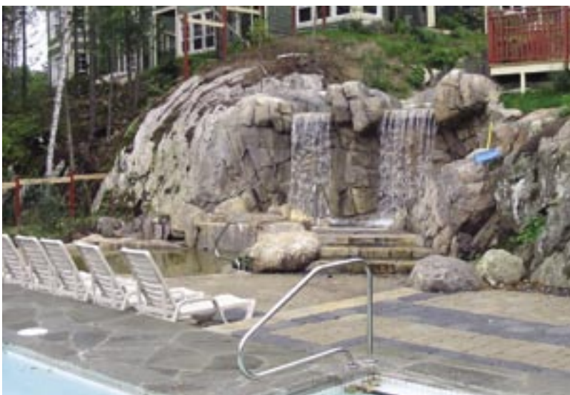
Fig. 8: Waterfall shot onto rock is natural looking and hardly distinguishable from natural rock
