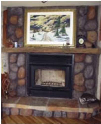
Fig. 2: A shotcreted fireplace
