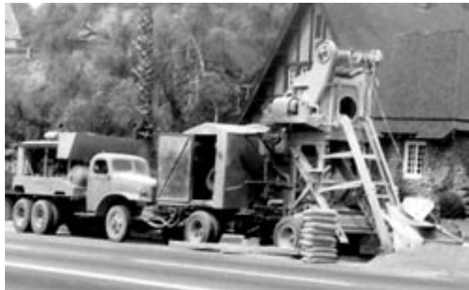
Fig. 4: Typical shotcrete rig used for structural work prior to the mid-1970s
