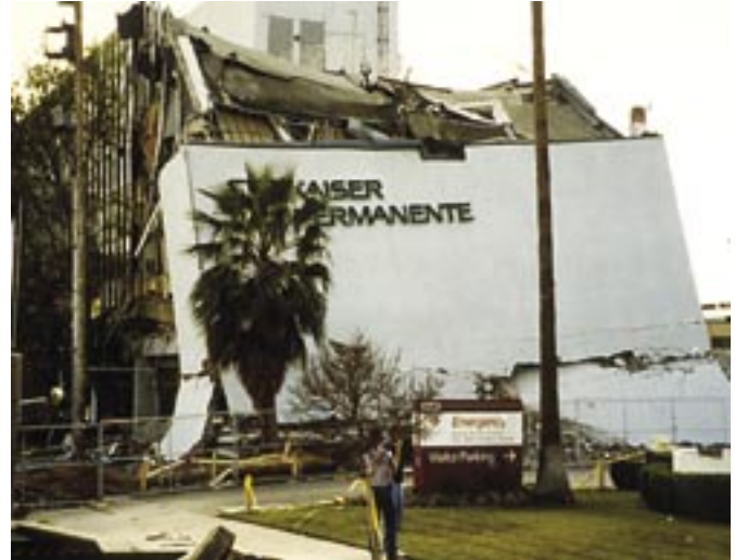
Fig. 9: Shotcrete overlay literally slid down like a curtain as building collapsed
