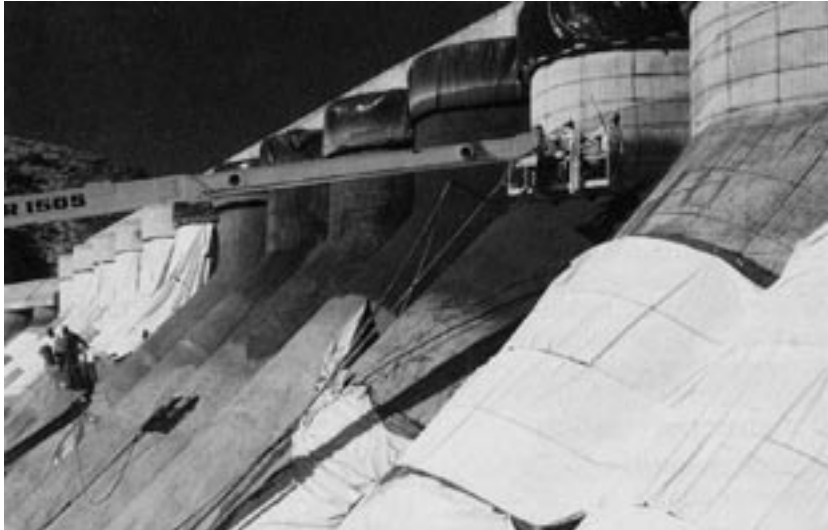
Fig. 8: General view of shotcrete repair with installed curing blankets
