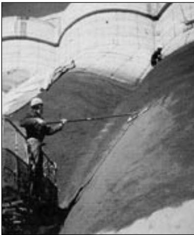
Fig. 7: Shotcrete finishing using a long-handled metal bullfloat
