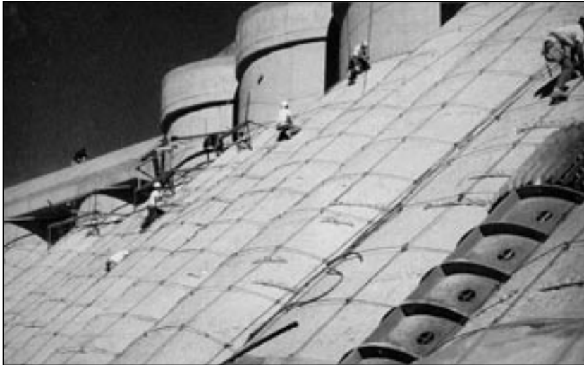
Fig. 6: Anchors and reinforcing steel installed on the face of the dam
