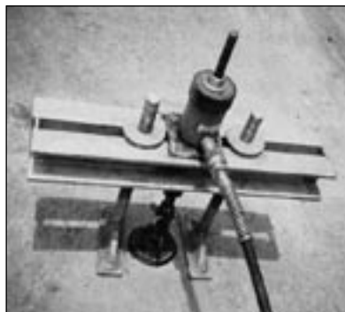
Fig. 4: Installed bond pull-off test apparatus
