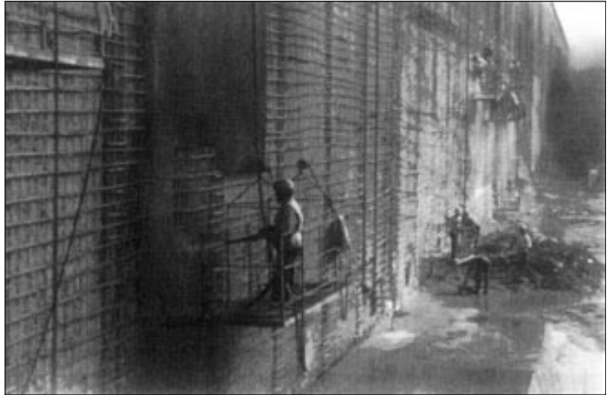
Fig. 4: Shotcreting in progress
