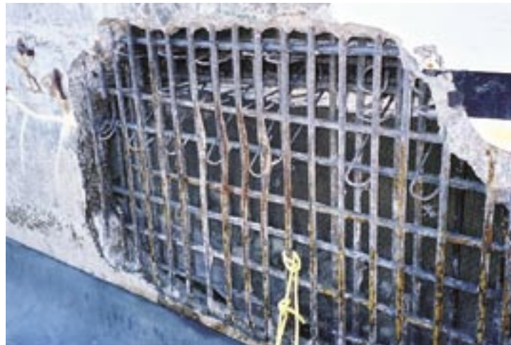
Fig. 4: Mesh forming used. Note the gaps around the edges
