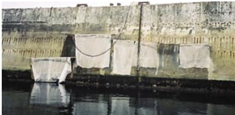
Fig. 8: The curing regime in place. Note the proximity of the waterline to some of the patches
