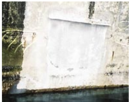
Fig. 9: The gutter used over the patches when rain was encountered
