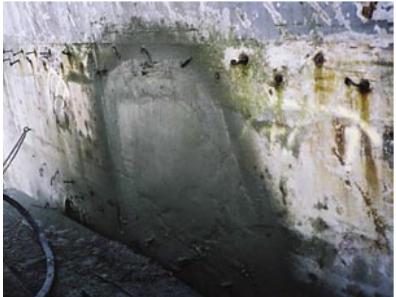
Fig. 7: The finished patch
