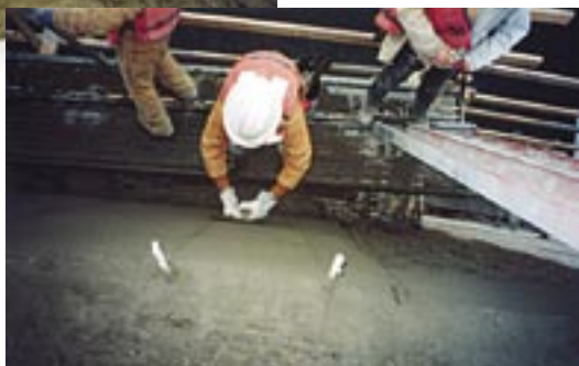
Final shaping to shoot wires
