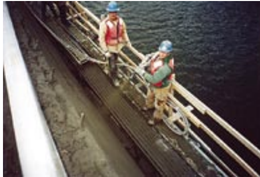
Wet-mix shotcrete application with less than 5% rebound
