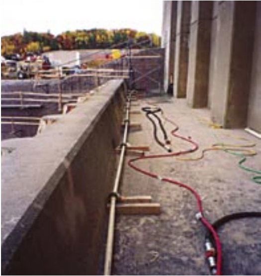
Shotcrete product pumped approximately 300 ft
