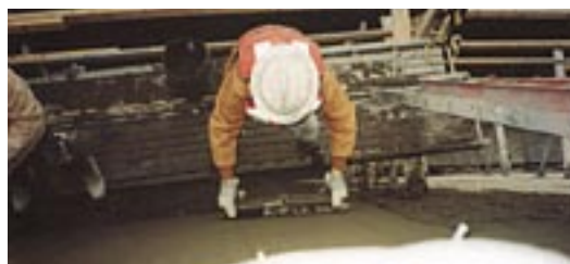
Light broom finish after surface shaping of shotcrete
