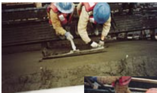
(left) Rough cutting to shoot wires with Fresno float
