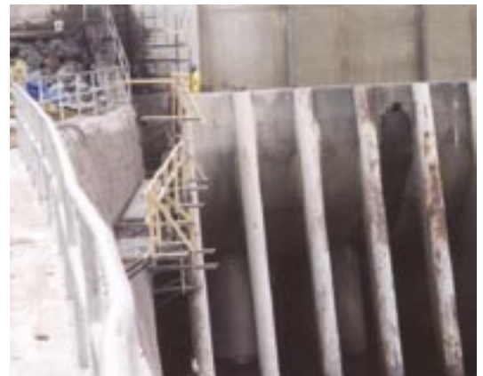
Access to dam area, with safety protection
