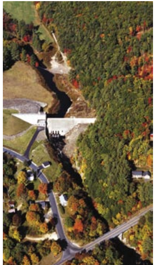
Fig. 2: Aerial view of Blackwater Dam
