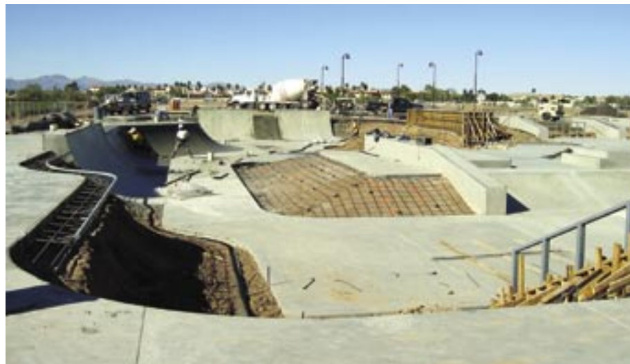
Finishing multiple wall sections after shotcrete application
