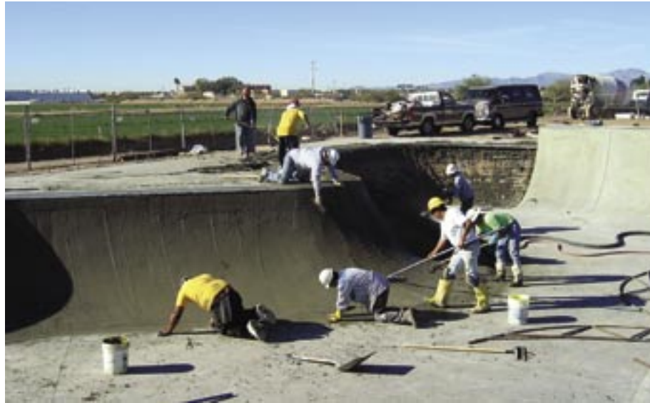
Trowel finishing a radius section at the skatepark
