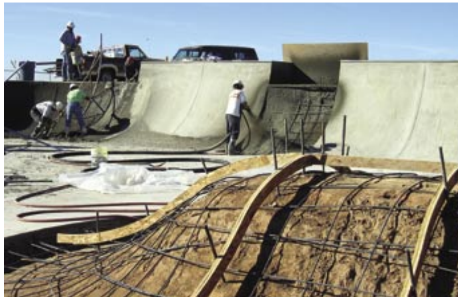
Shooting a vertical wall section
