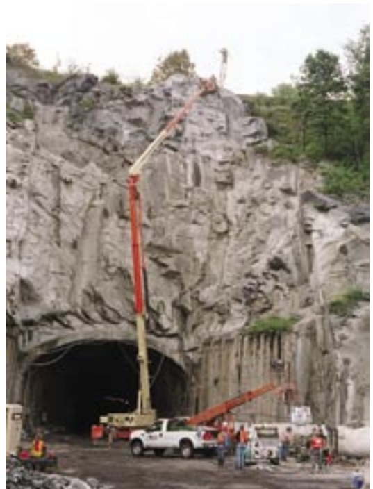
East Portal sculpted shotcrete application
