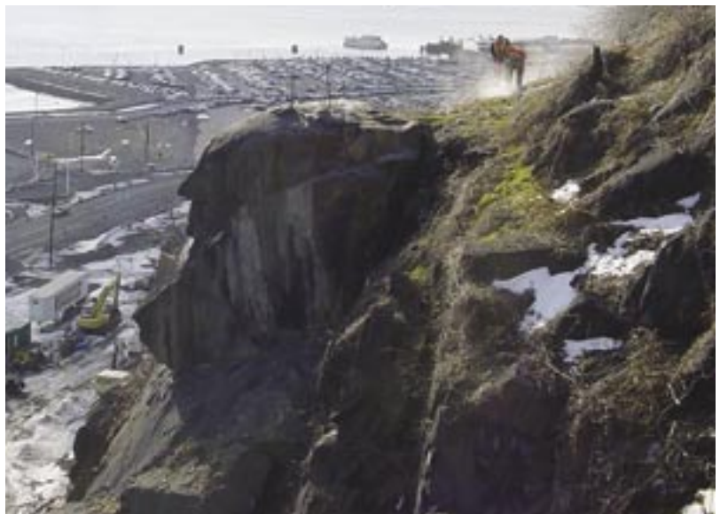
Gorilla's head formation above Weehawken Tunnel East Portal
