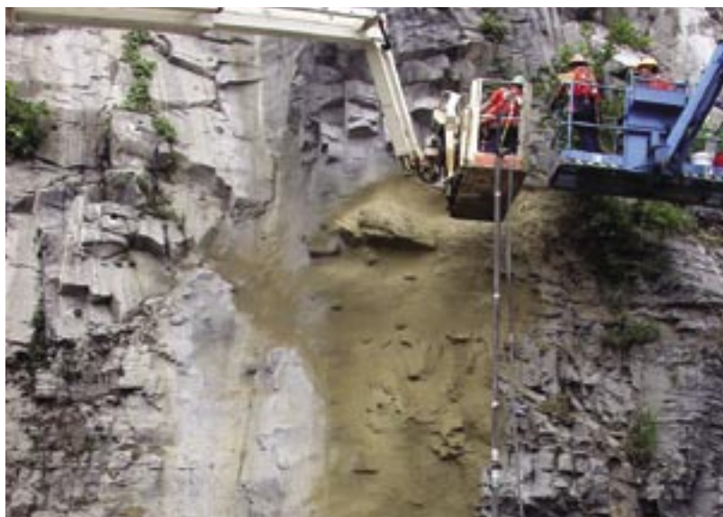
Test section for approval of sculpting
