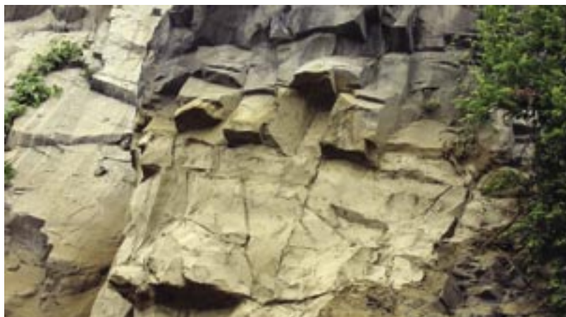
Rough finish of test area
