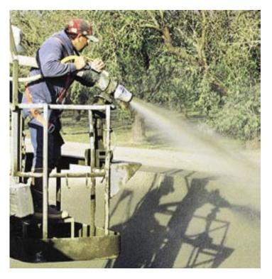
directions provided when introducing the fibers into the mixing system in order to achieve uniform distribution. Where safety is an issue, a flash coat of non-fiber-reinforced shotcrete can be applied over steel fiber-reinforced shotcrete to cover the exposed ends of the steel fiber.
