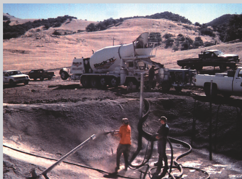
Waterproofing repairs underway at the Talent Irrigation District grass carp pond
