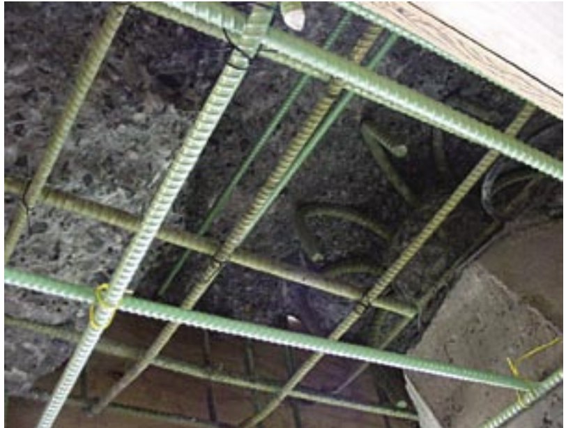
Fig. 2: Prepared spalled area ready for shotcreting
