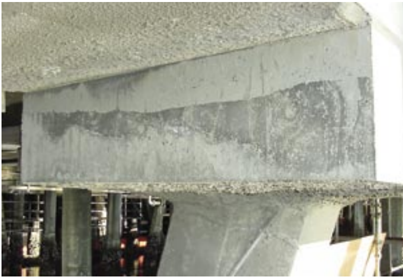
Fig. 3: Shotcrete repaired pile cap
