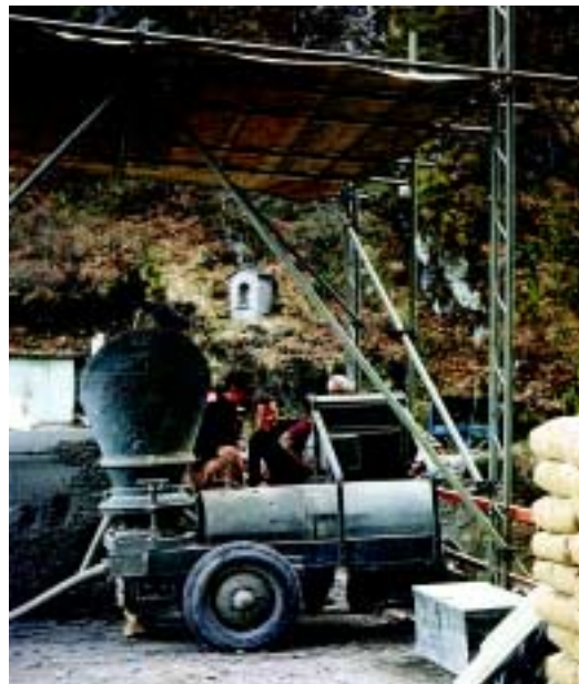
Figure 4: American rotating-barrel gun (Jetcreter).
