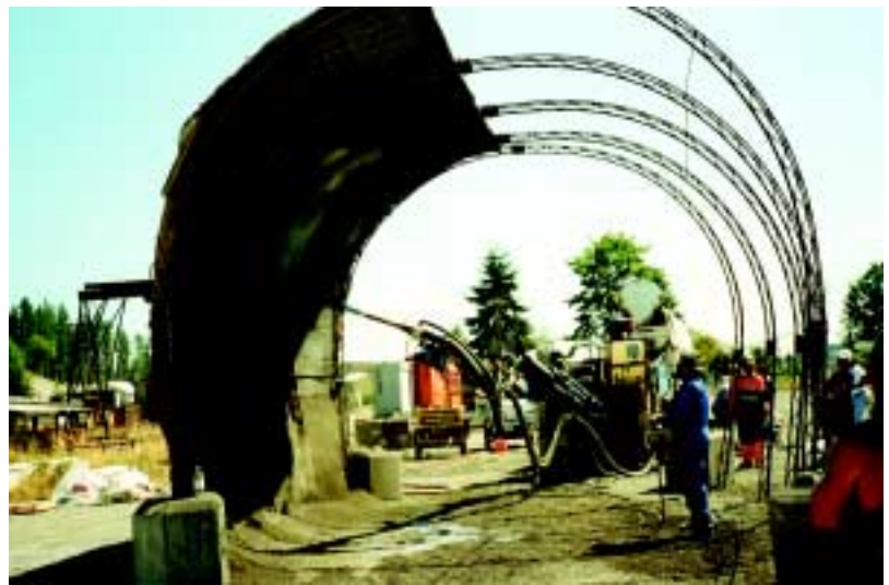
Figure 5: Meyco 2.5 in. (63.5 mm) nozzle/Seattle Rock Mechanics Demo
