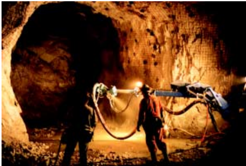
Figure 7: Ground support/Henderson Mine
