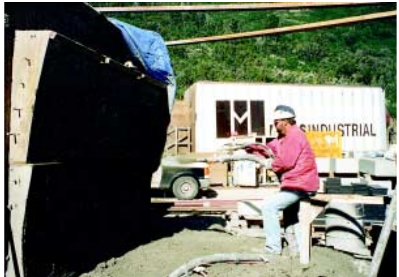
Figure 1: Shooting test panels, bobsled and luge track, Park City, UT
