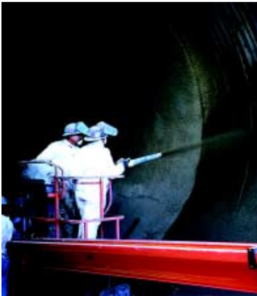
Figure 4: Meyco 2 in. (50 mm) nozzle (Photo courtesy of George Yogy)
