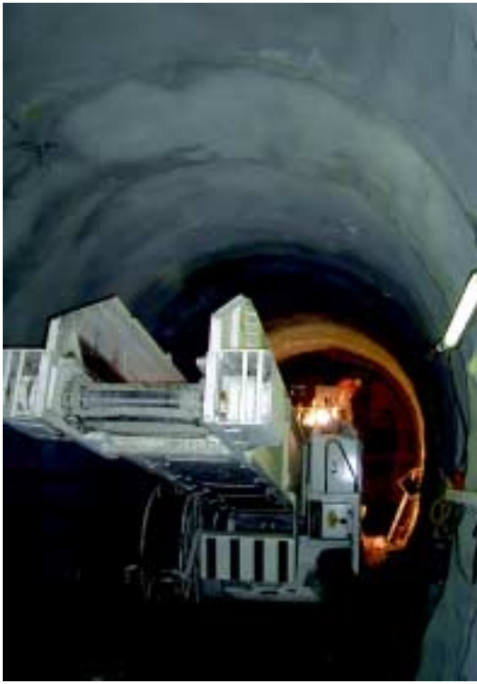
Figure 2: After excavation by the ITC-Schaeff, tunnellers erect lattice girders ahead of immediate shotcrete support in the central pilot heading through the 340 m (1115 ft) section of unconsolidated material in the west portal zone.
