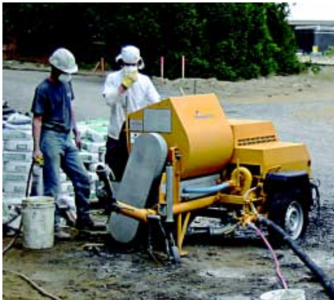
Figure 2: Wet-mix shotcrete pump.
