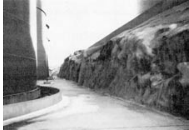
Fig. 8: Portion of rock surface stabilized at Brofjorden Refinery, Sweden.
