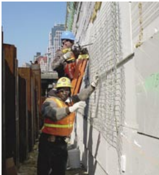
Fig. 5: Olympic fasteners are used to fasten wire mesh to EPS block.
