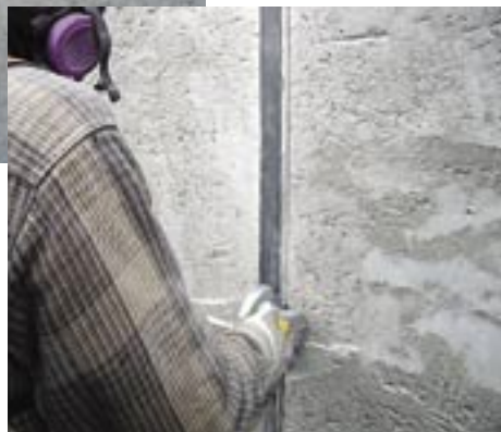
Fig. 8: Steel is attached to shotcrete face to ensure straight edges on expansion joints.
