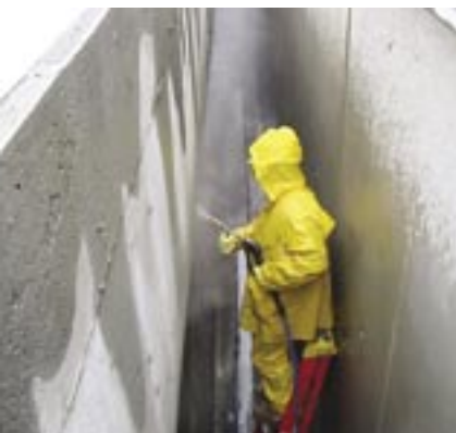
Fig. 9: Pressure washing was performed before application of concrete refacing.
