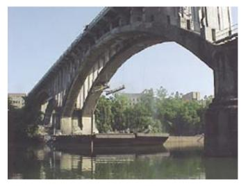
specification called for form and pour repairs on the piers. The use of dry-mix shotcrete resulted in cost savings and reduced time spent on repairs while providing a high-quality repair solution. The shotcrete portion of the project was a major part of the bridge restoration.
