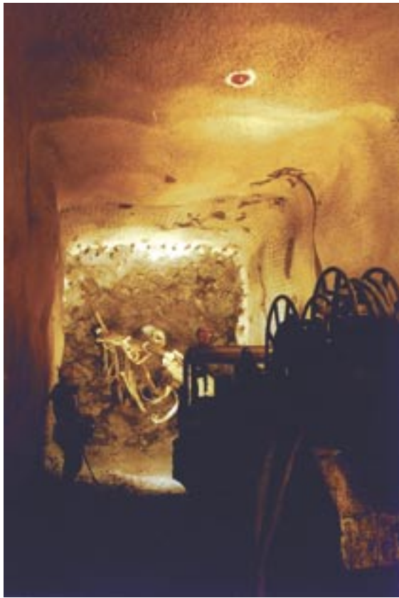
In-cycle shotcrete application at Perseverance Mine.
