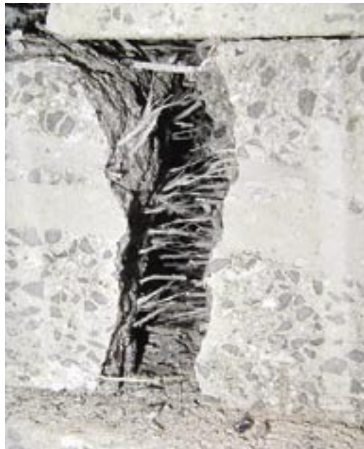
The round panel test has highlighted the importance of fiber behavior. It is essential that fibers fail in pullout mode as shown in this photograph. If the fibers snap before pulling out, a fast brittle failure occurs. This must be avoided in a mining environment.
