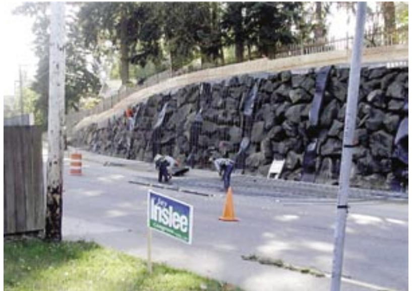
Figure 5: Fractured fin forms.
