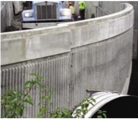
Figure 4: Fractured fin on a radius.
