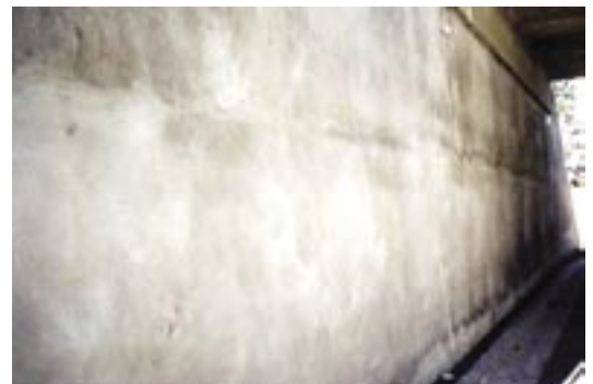
Figure 3: Nonpigmented rubber float finish with top-down construction.
