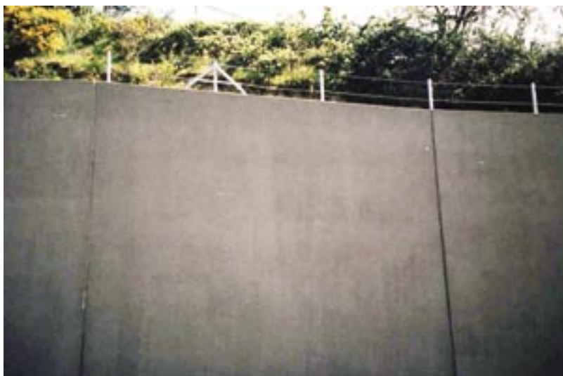
Figure 2: Vertical broom finish with pigmented sealer.
