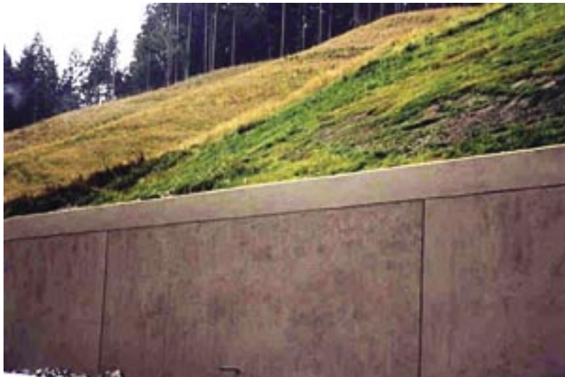
Figure 1: Wood float with pigmented sealer.
